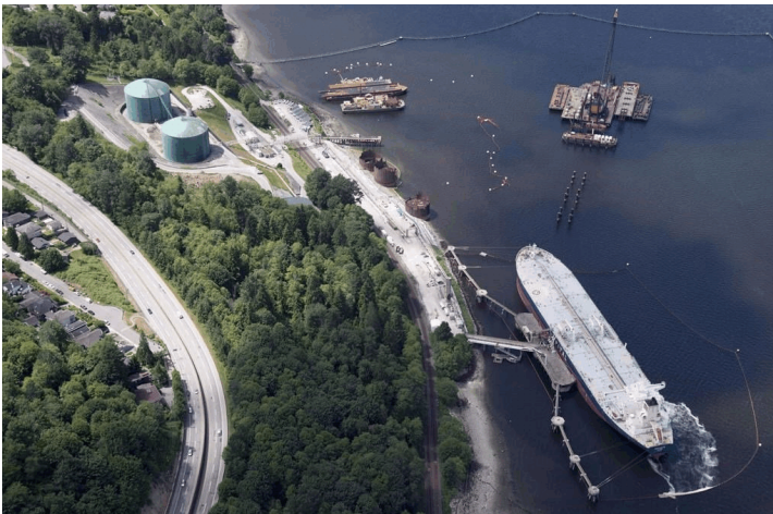
Figure 4: The Aristoklis at the Kinder Morgan Westridge dock on May 29, 2018. Some of the construction for the planned new docks is also seen. The two green tanks are for storing imported jet fuel. Photo by The Canadian Press/Jonathan_Hayward.
